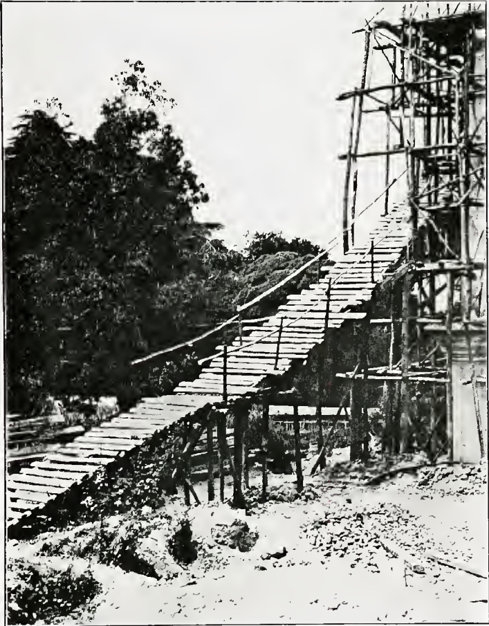
PORTUGUESE SCAFFOLD LADDER: BUSSACO
